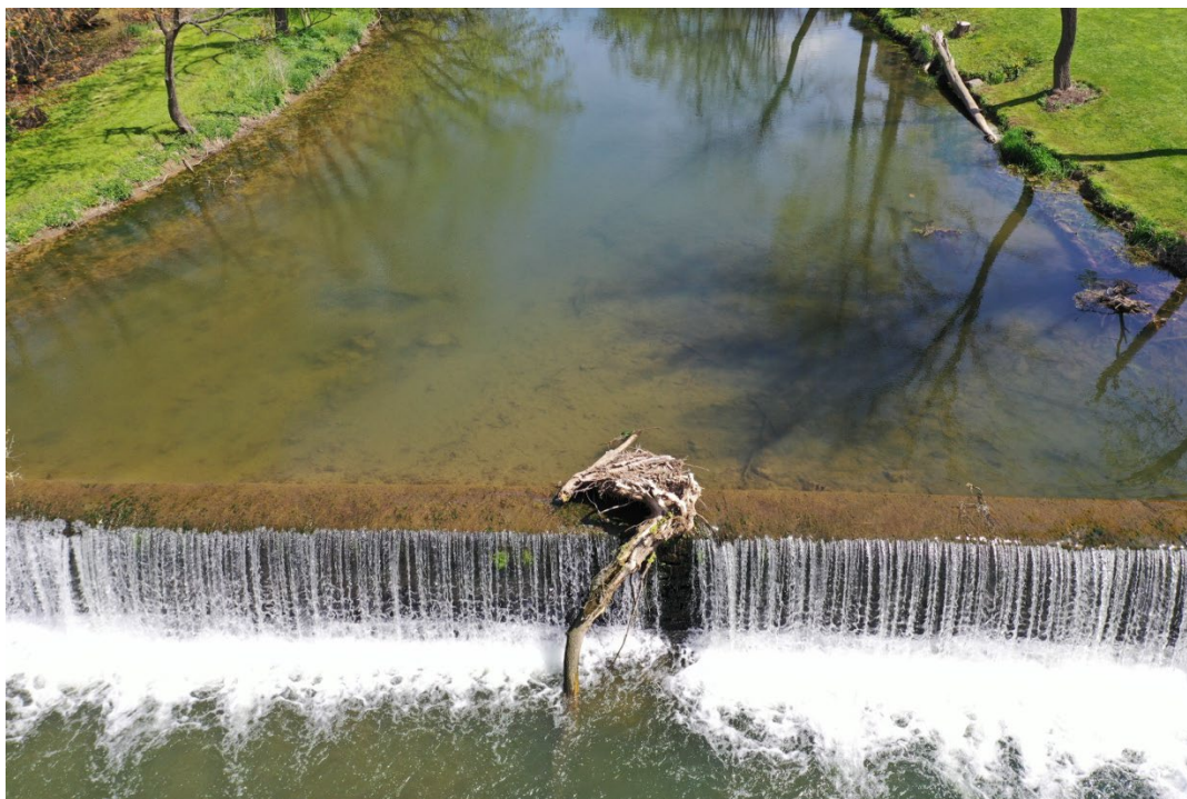
Figure 1: View of Roller Mill Dam with stored sediment.
